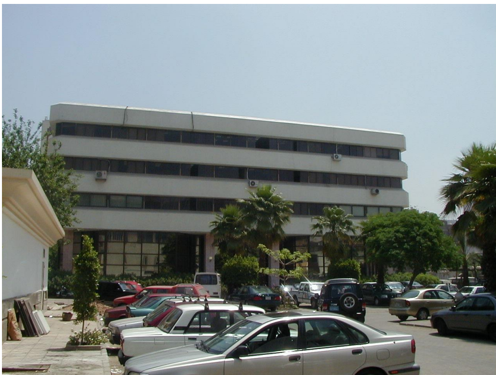
Training Centre of HBRC, where the headquarter of UTI is located, Giza, Egypt.
