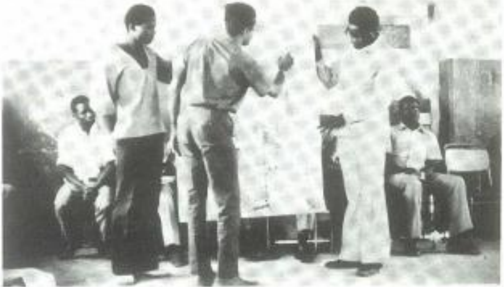
Plate 3.3 The Road Planning Group's proposals are put down on paper and discussed before a final commitment is made. Here they are shown being presented by the chief engineer, the architect and the chief community development officer.
