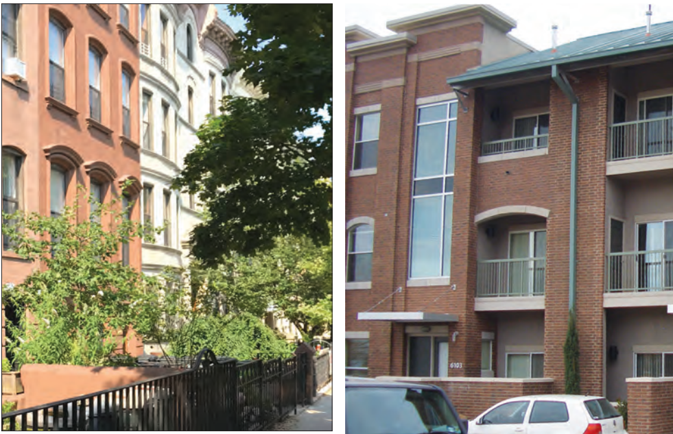
Figure 7: On the left, an old multi-story townhouse and, on the right, a new townhouse with no stoop for privacy from the sidewalk level.
