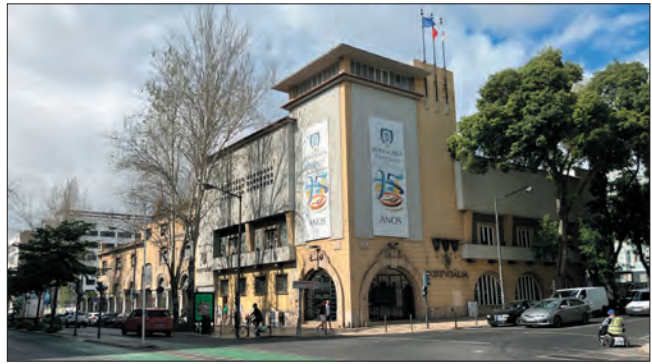
Figure 5: Corner of Avenida Almirante Reis and Rua Pascoal de Melo. The Portugalia restaurant and, on the left, the deteriorated historic building. (photo: V. del Rio)
