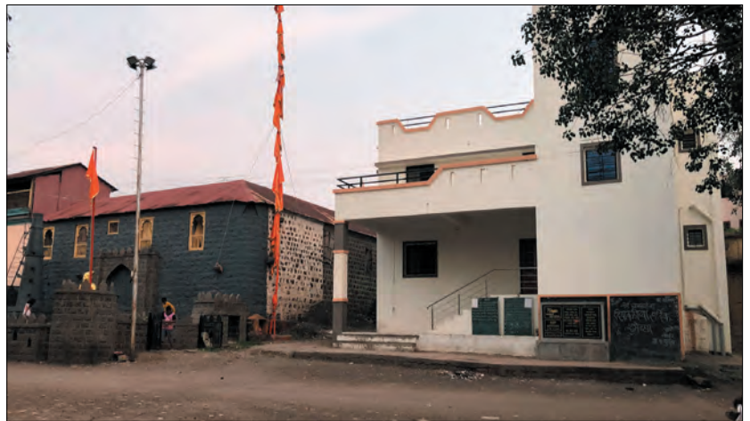
Figure 8: The new village hall is two-story, sturdy, and built of cement concrete plastered white.
